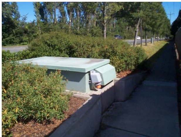
Access Concealed Through Grade
