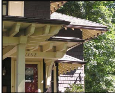
Figure 15.39.320I Example of rafter tails.
