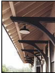
Figure 15.39.320H Example of deep roof overhangs and brackets.
