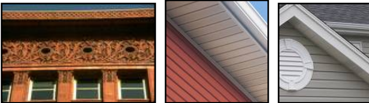
Figure 15.39.320K Examples of cornice, soffit and fascia details.
