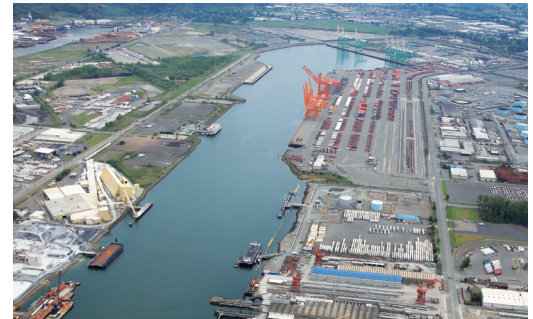
Relieves traffic congestion and completed a critical freight link between the Ports of Tacoma and Seattle.
