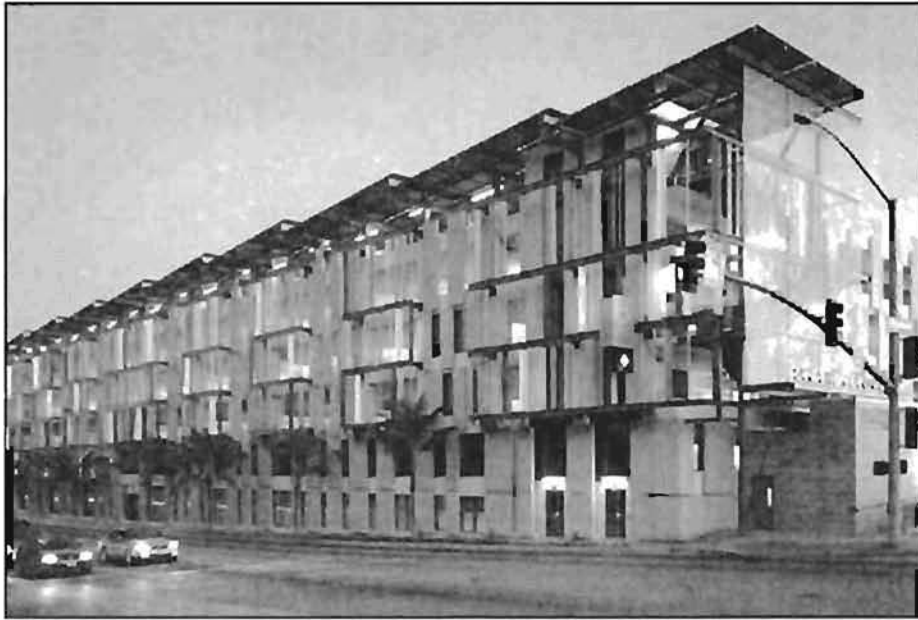
Figure 15.35.1056C – Example of upper floor screening using window like openings and other screening materials.
