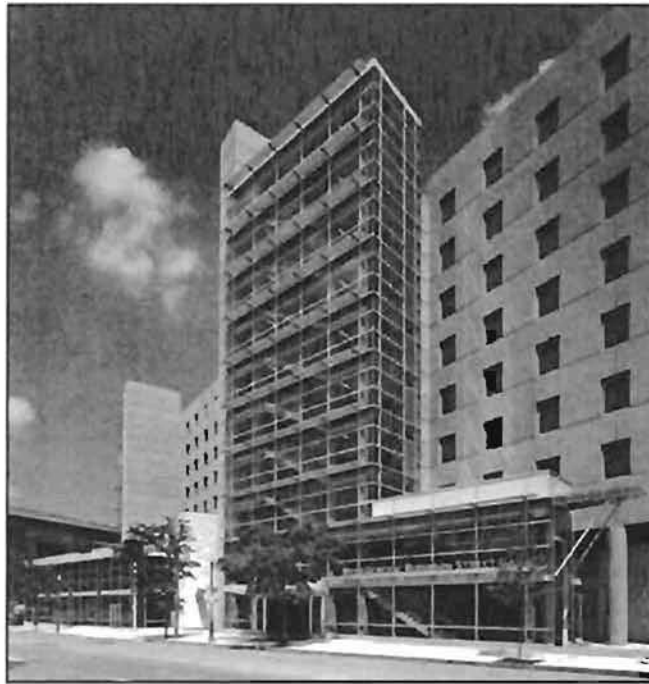
Figure 15.35.1056B(1) – Glazed stair tower as a roof/top floor focal point.
