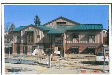
Update: Foundation work continuing. Siding being installed. Apparatus bays now in framing.
