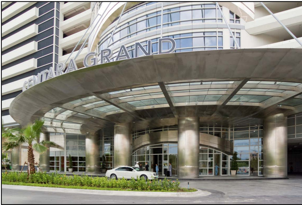
Figure 15.35.1051C – Pedestrian entry with a covering and a distinctive architectural element.
