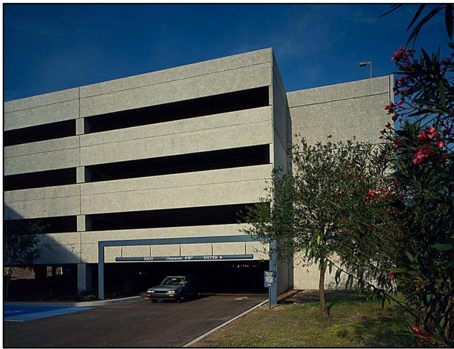
Figure 15.35.1051F(3) – Example of undesirable building materials – bare concrete as predominate façade treatment.
