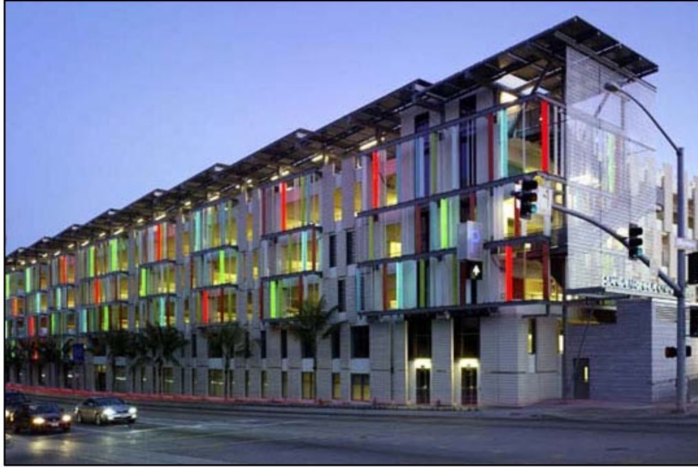
Figure 15.35.1053B – Example of upper floor screening using window like openings and other screening materials.
