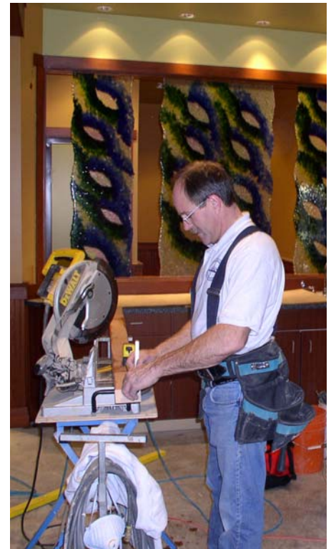
Pat Patterson, Facilities Director, working on the new Senior Center addition.
