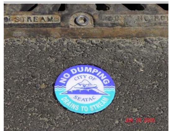
The City uses a Catch Basin Curb Marker Program to partner with schools and volunteer organizations to mark the storm drain inlets and catch basins.
