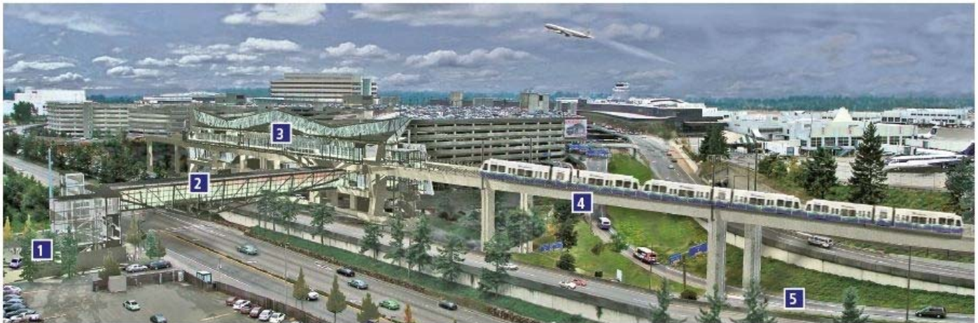
Sound Transit's light rail project at Seattle-Tacoma Airport: 1. pick-up/drop-off area; 2. pedestrian bridge; 3. SeaTac/Airport Station; 4. elevated guideway; 5. airport expressway relocation.
