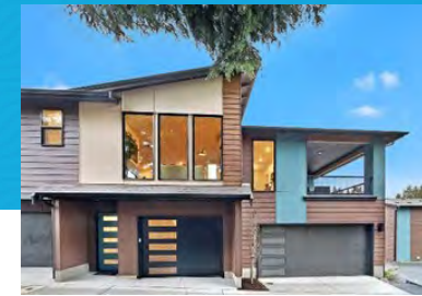
COTTAGE HOUSING DEVELOPMENT Velorum, 10 units, Mountlake Terrace
