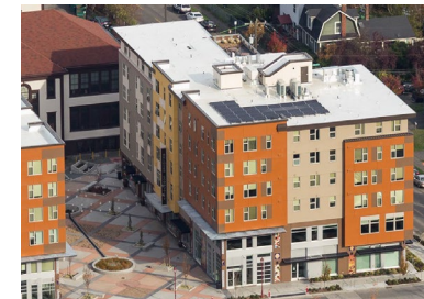
MIXED USE APARTMENTS Plaza Roberto Maestas Affordable Housing Beacon Hill, Seattle
