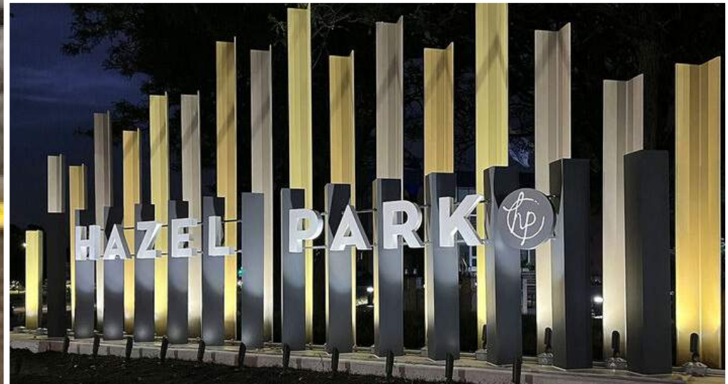
Uplighting between layers
