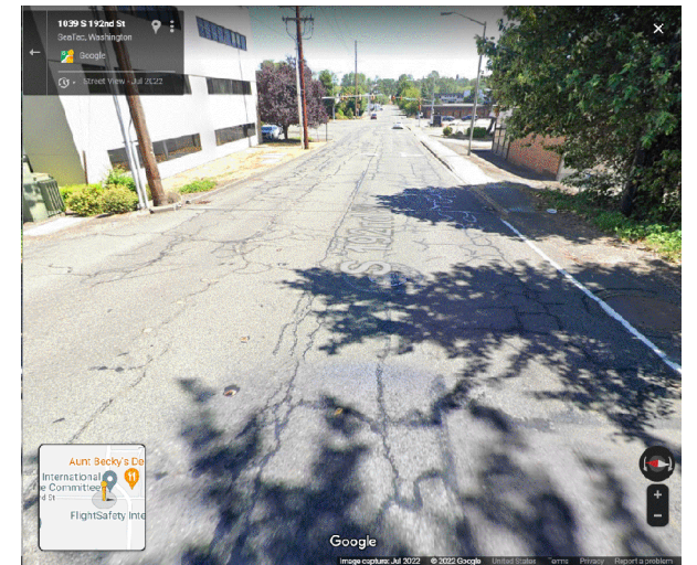
EXISTING S192ND VIEW AT EAST R/W LINE LOOKING EAST
