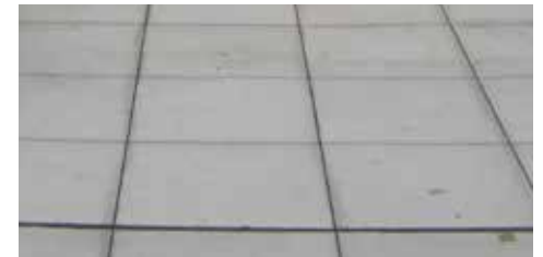
2x2 scored cement concrete sidewalk
