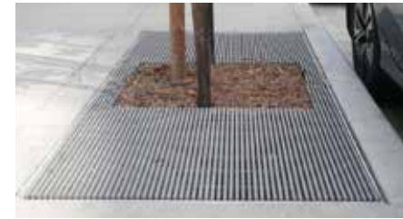
tree grates with breakaway opening, ADA compliant, heel proof
