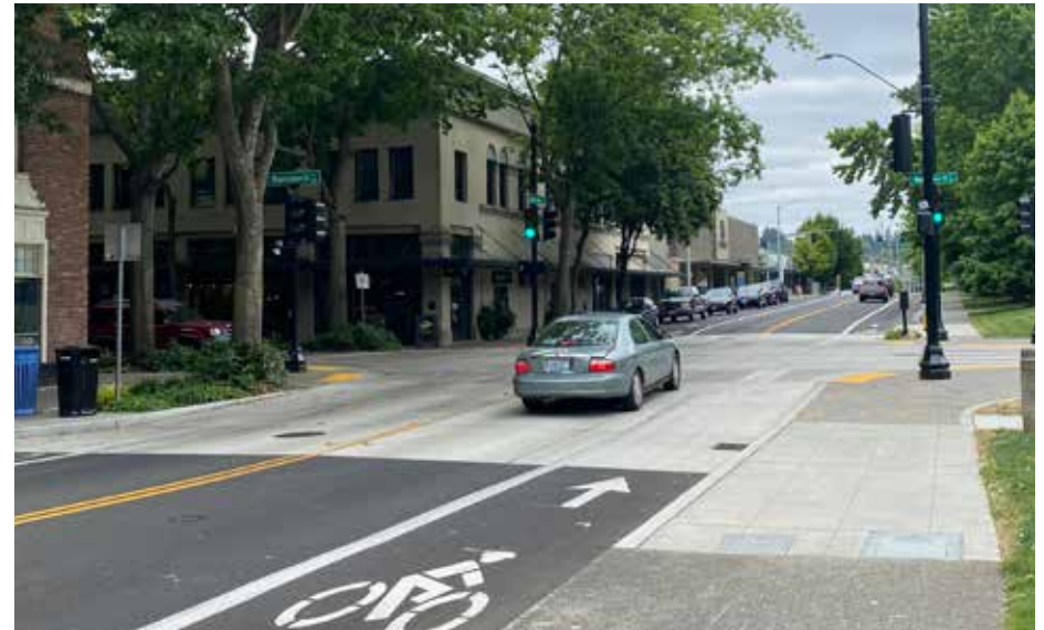
Photo example of raised concrete intersection
