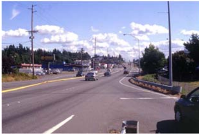
Figure 8: International Boulevard (SR 99) Toward South End of Future SR 509.
