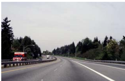
Figure 26: Existing SR 509 near 128th Street.
