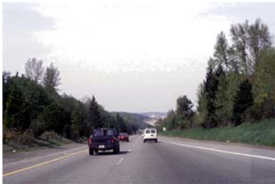
Figure 25: Existing SR 509 Northbound Approaching the Duwamish Valley.
