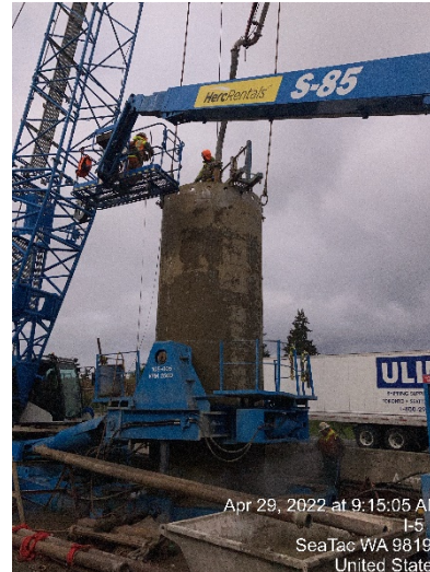
NBCD Bridge Pier 3 Shaft, SeaTac
