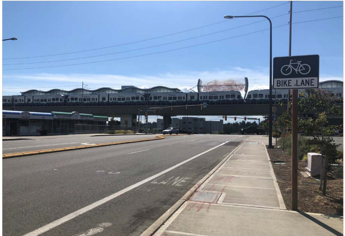
BIKE LANE ON SOUTH 200 TH STREET FACING WEST TOWARDS ANGLE LAKE STATION
