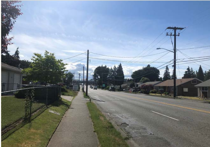
NARROW SIDEWALKS ON RESIDENTIAL SEGMENT OF SOUTH 200 TH STREET
