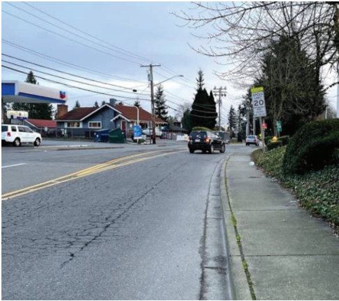
FIGURE 6: FACING SOUTHBOUND ON MILITARY RD S.
