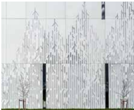
decorative concrete wall treatment w/ engraving finish
