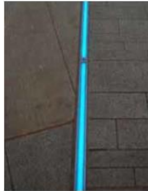
linear pavement lighting
