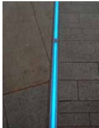
linear pavement lighting
