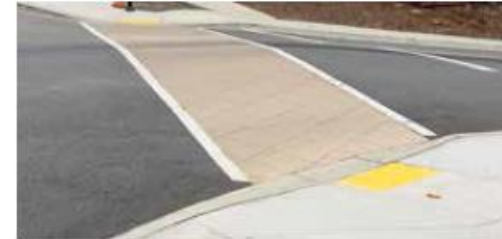
2x2 scored integral colored cement concrete crosswalk
