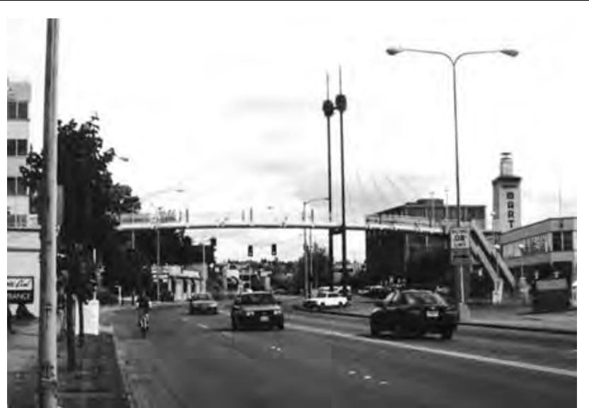
Pedestrian bridges can be designed to enhance the streetscape and create a sense of place along a busy road corridor.
