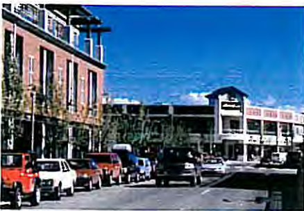
Buildings are distinguished by strong details and an attention to form.
