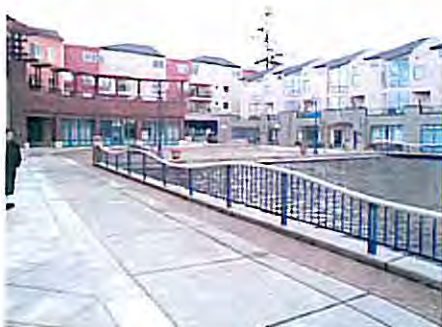
The promenade along the lake creates the major retail face.
