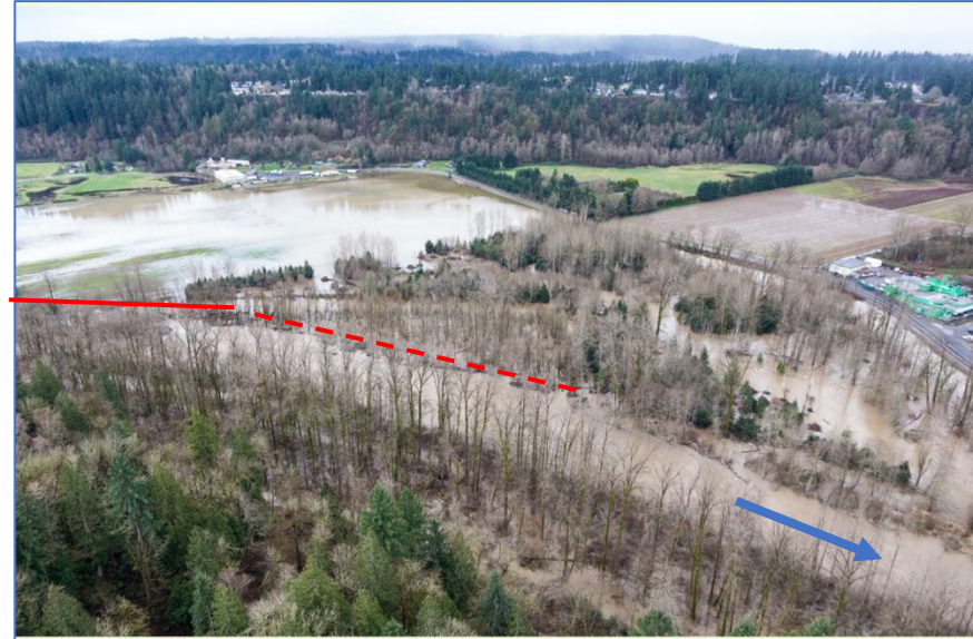
Porter Levee Setback
