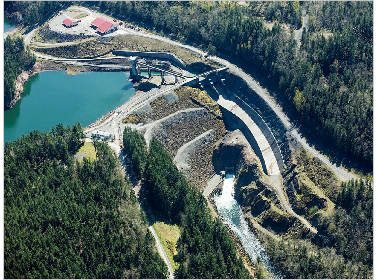
Howard Hansen Dam Fish Passage
