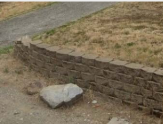
Retaining wall at residence at 17342 32 nd Avenue South
