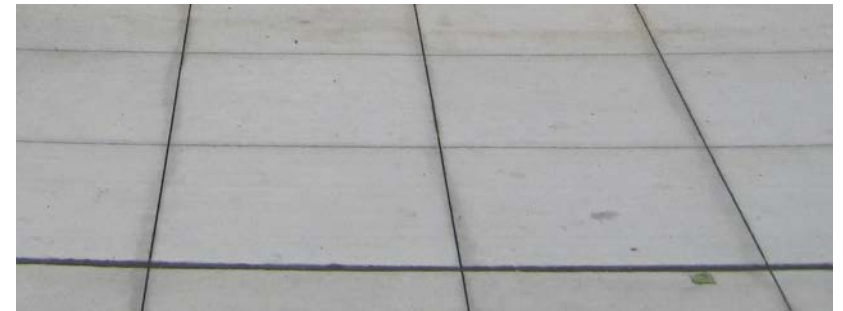
2x2 scored cement concrete sidewalk
