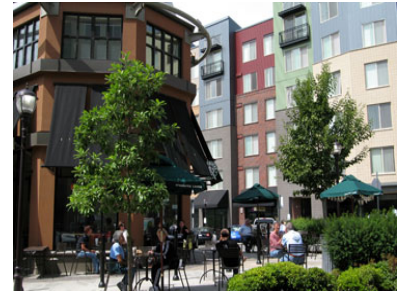
Figure 59. Example of unified landscaping, lighting, sidewalk and street furniture design in Kirkland, WA.
