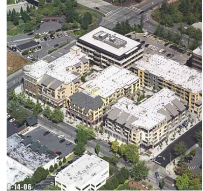
Figure 26. The Island Square project is a significant mixed use development that is contributing to the revitalization of downtown Mercer Island, WA.
