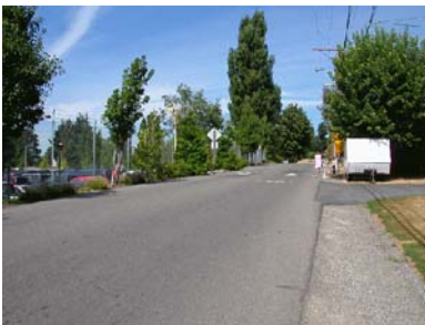
Figure 19. Gravel shoulder and speed bumps along 32 nd Ave S north of S. 176 th St.
