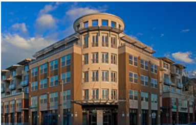
Figure 57. The Island Square development in Mercer Island, WA.
