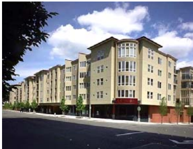
Figure 58. Retail/commercial space with residential above in Bellevue, WA.
