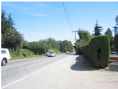
Figure 18. Gravel shoulder (to be paved) along S. 154 th St.
