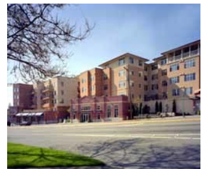
Figure 54. Tera Apartments in downtown Kirkland, WA are a good example of mixed use development.
