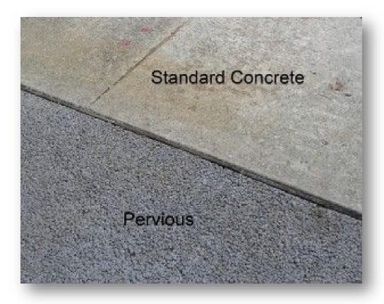
The photos above show pervious concrete, often referred to as "popcorn" concrete, adjacent to impervious brush finished concrete. The porous nature of the pervious concrete allows water to pass through the material rather than runoff; use of this type of concrete helps projects reduce stormwater runoff and meet regulatory requirements.
