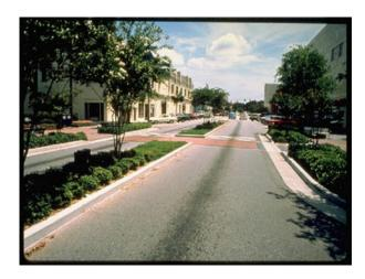
These techniques provide a flexible way to take back space from the street for non-motor-vehicle uses. Traditional traffic engineering calls for 12- to 13-foot lanes, citing "traffic safety" standards – but newer evidence shows that lanes as narrow as nine feet can still be safe for driving.
