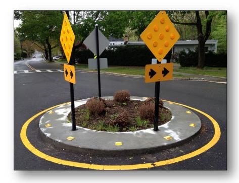
Essentially "mini-roundabouts" designed for small intersections, often used to slow traffic from a wide street into a smaller local street. Traffic circles:
