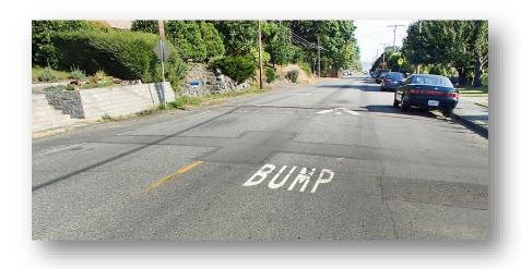
These devices reduce speed by introducing modest up-and-down changes in the level of the street, thereby requiring drivers to decelerate.
