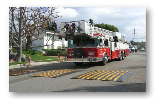
It is important to highlight road humps, speed tables and cushions with clear markings to alert approaching drivers. This can be accomplished by: painting words and symbols directly on the street; changing the texture of the street surface; or using signage (the word "Bump" instead of "Hump" is a standard approach thought to effectively put drivers on the alert).
