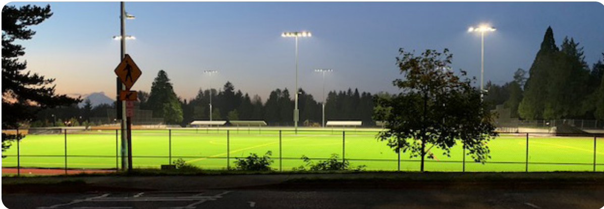
North SeaTac Park Soccer Field Renovations 2020
