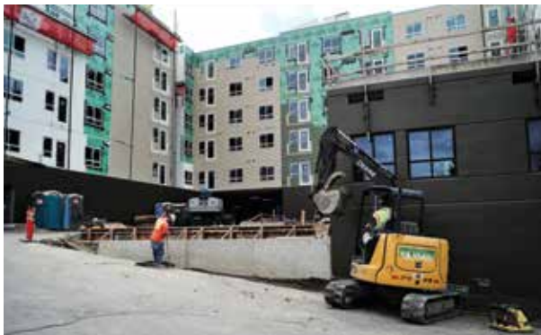
VINTAGE SENIOR HOUSING CONSTRUCTION
