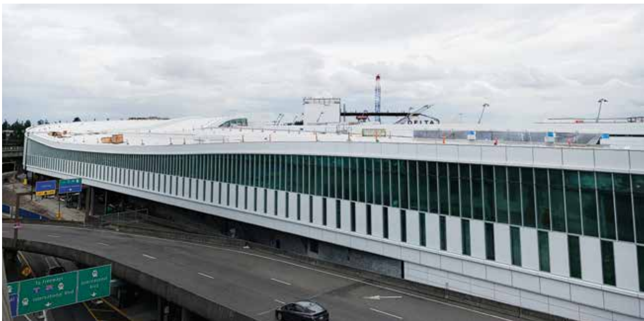
NEW SEA-TAC AIRPORT INTERNATIONAL ARRIVALS FACILITY
