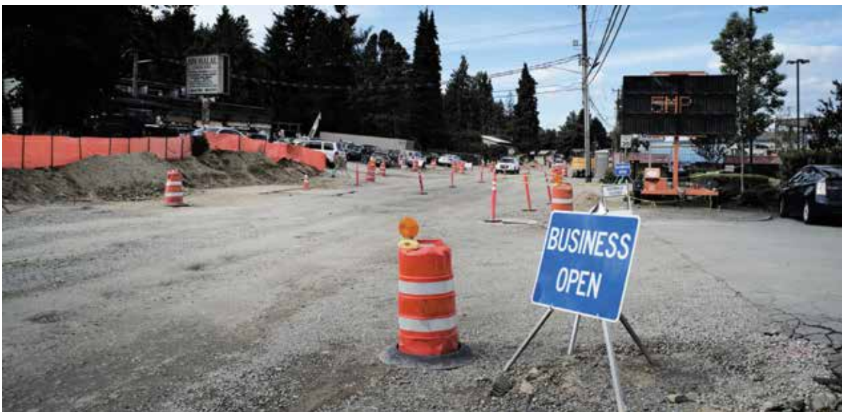
CONSTRUCTION ON MILITARY ROAD S. AND 152ND STREET
