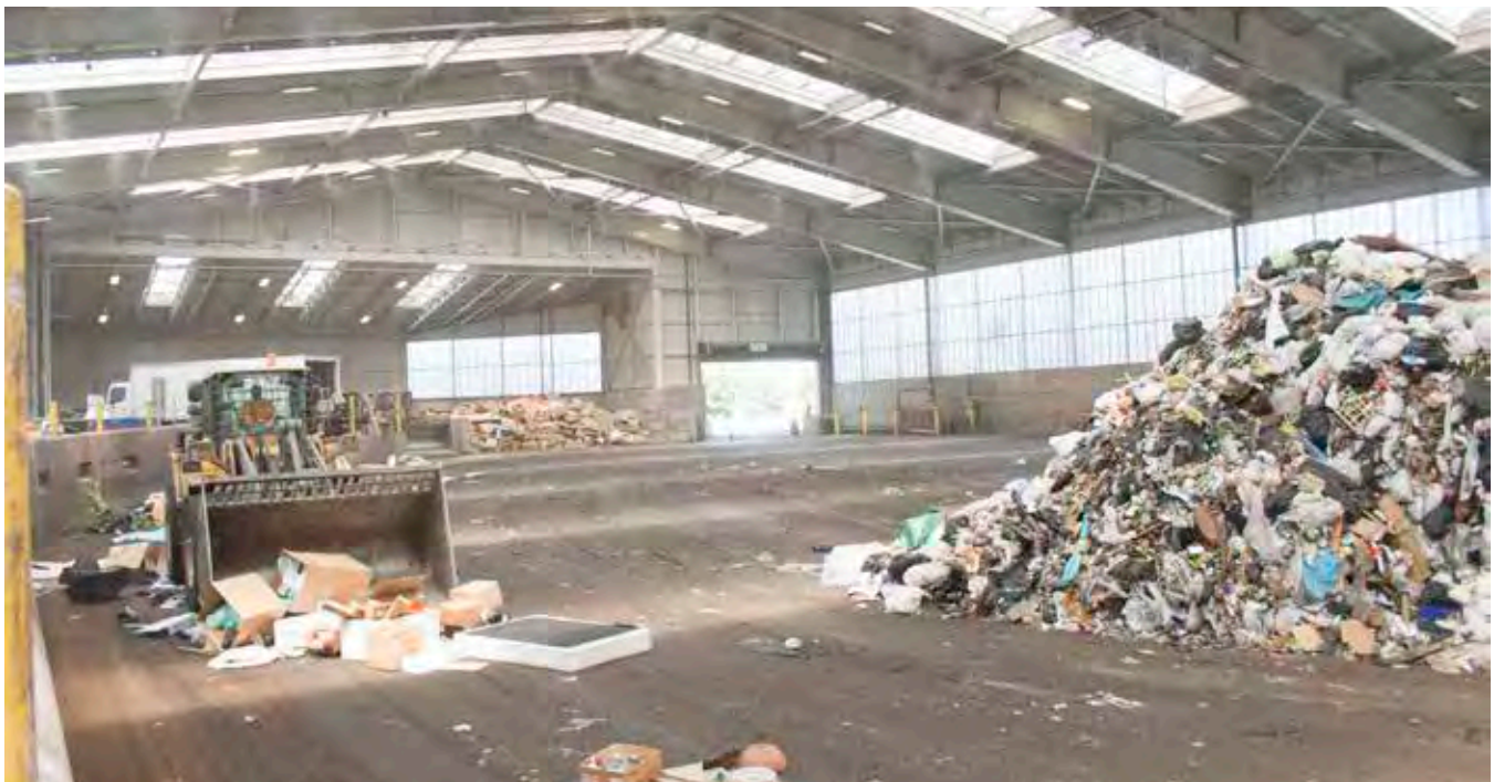
Bow Lake Recycling and Transfer Station
