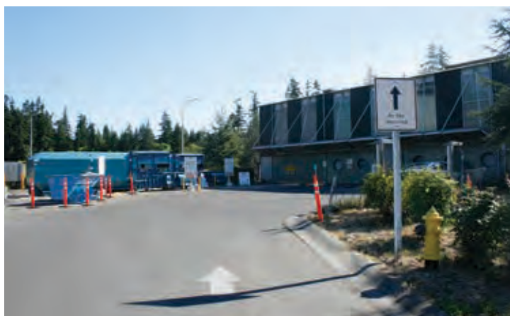
The Vashon Recycling and Transfer Station
