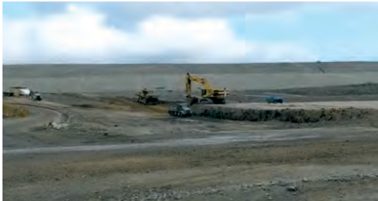
Developing a new area requires extensive excavation and preparation
