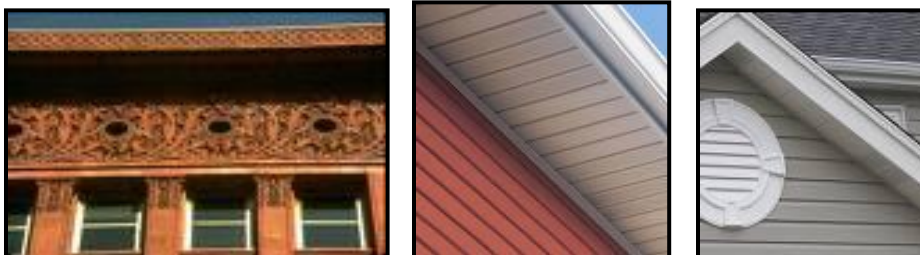
Figure 15.525.320K. EXAMPLES OF CORNICE, SOFFIT AND FASCIA DETAILS.
