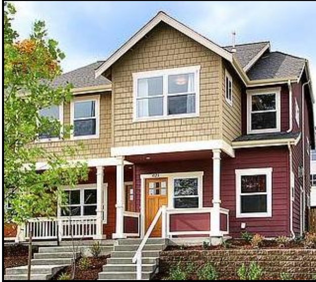
Figure 15.525.310A CLEARLY DEFINED MAIN ENTRY WITH WEATHER PROTECTION AND VARIOUS ARCHITECTURAL DESIGN ELEMENTS
