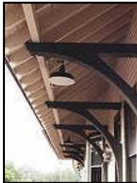
Figure 15.525.320H. EXAMPLE OF DEEP ROOF OVERHANGS AND BRACKETS.
