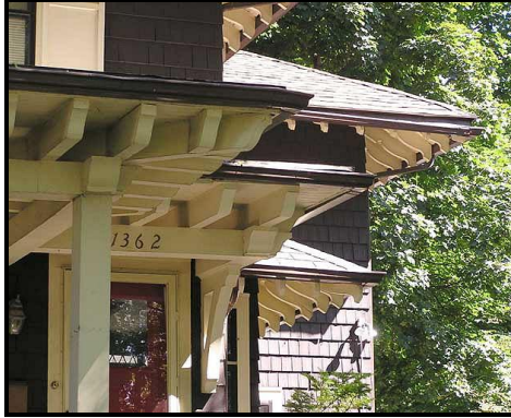
Figure 15.525.320I. EXAMPLE OF RAFTER TAILS.
