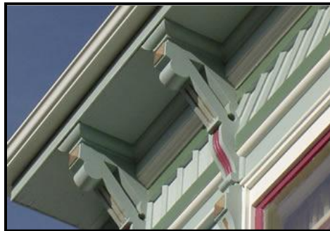
Figure 15.525.320J. EXAMPLE OF CORBELS (WHICH ARE GENERALLY THICKER THAN BRACKETS).
