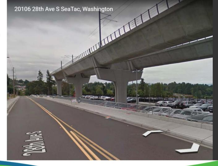
Future FWLE Guideway and Hwy 509 alignment Typical guideway width – approx. 30' Height to bottom of guideway at crossing – approx. 32 - 38'
