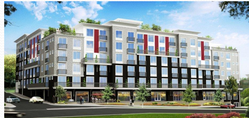
Project on SR99 in Shoreline
