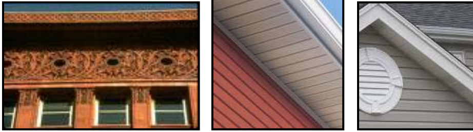
Figure 15.52539.320K Examples of cornice, soffit and fascia details.
