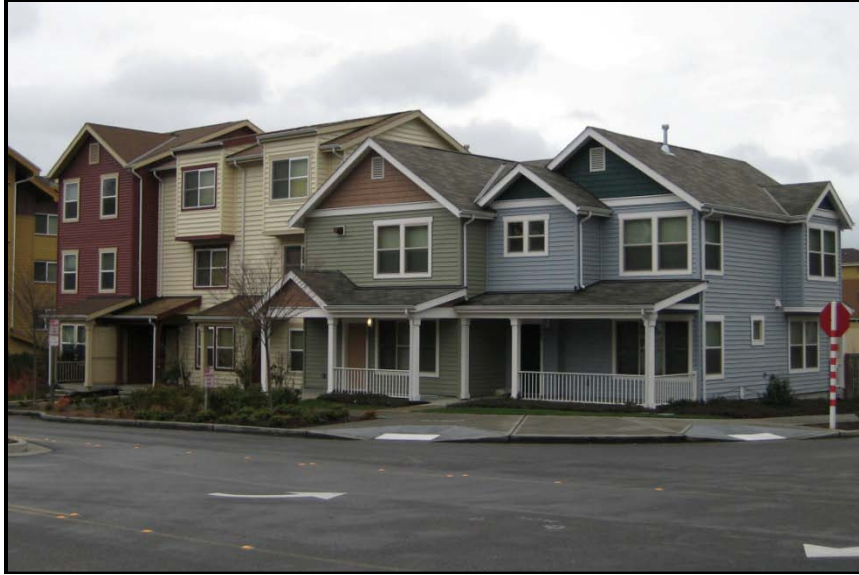
Figure 15.52539.220A Example of units oriented to the street.
