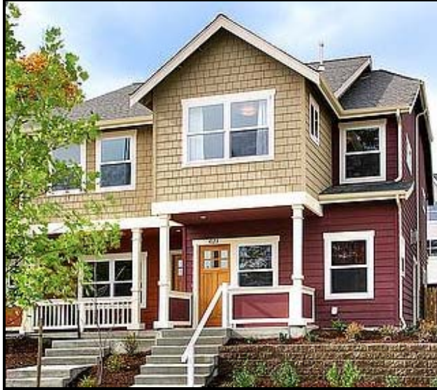
Figure 15.52539.310A Clearly defined main entry with weather protection and various architectural design elements
