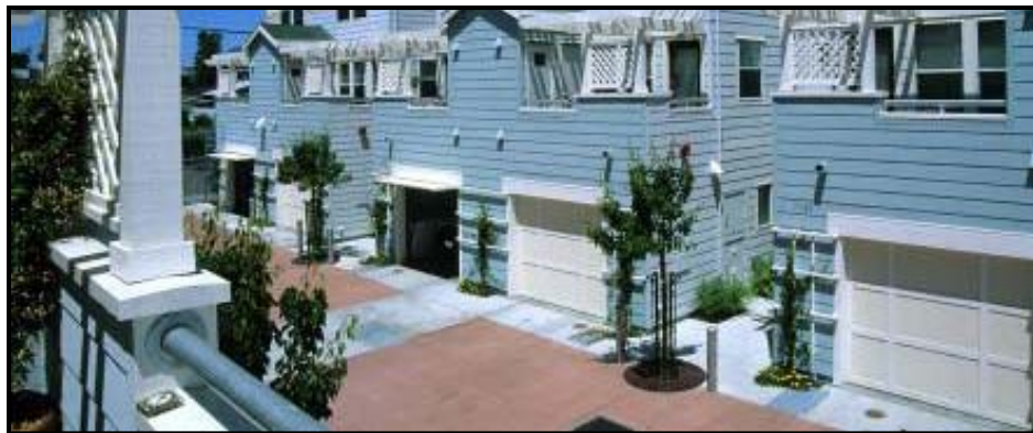
Figure 15.52539.240C Example of auto court constructed with scored and dyed concrete.
