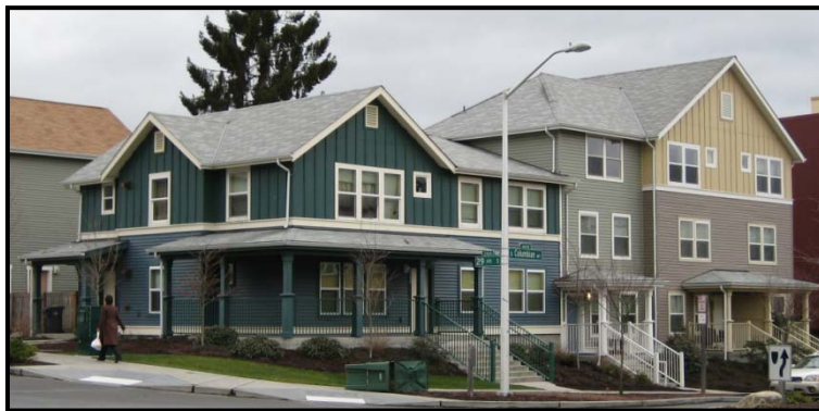
Figure 15.52539.320F Example of vertical and horizontal changes in rooflines and variations in roof forms.
