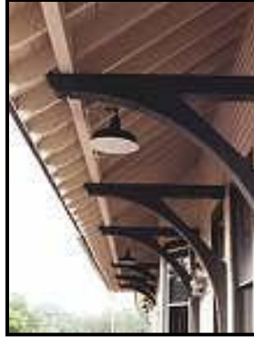
Figure 15.52539.320H Example of deep roof overhangs and brackets.
