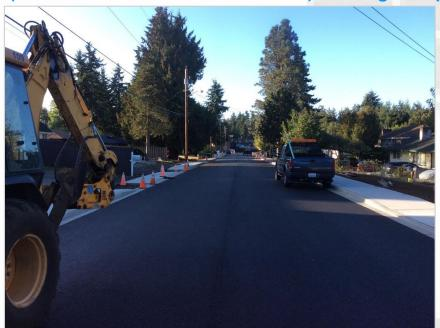
Construction is nearing completion for this project. Installation of sidewalk and paving were completed a few weeks ago. This week's work included hydroseeding to establish grass, restoration of disturbed areas, fence and signage installation, and driveway paving.
