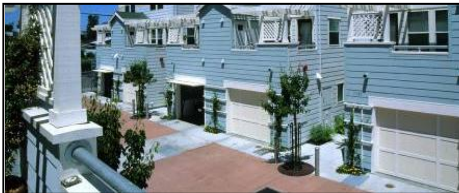
Figure 15.39.240C Example of auto court constructed with scored and dyed concrete.
