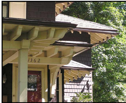
Figure 15.39.3201 Example of rafter tails.
