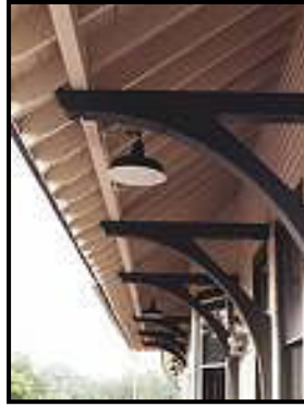
Figure 15.39.320H Example of deep roof overhangs and brackets.
