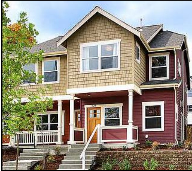
Figure 15.39.310A Clearly defined main entry with weather protection and various architectural design elements
