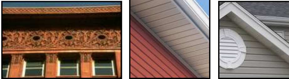
Figure 15.39.320K Examples of cornice, soffit and fascia details.
