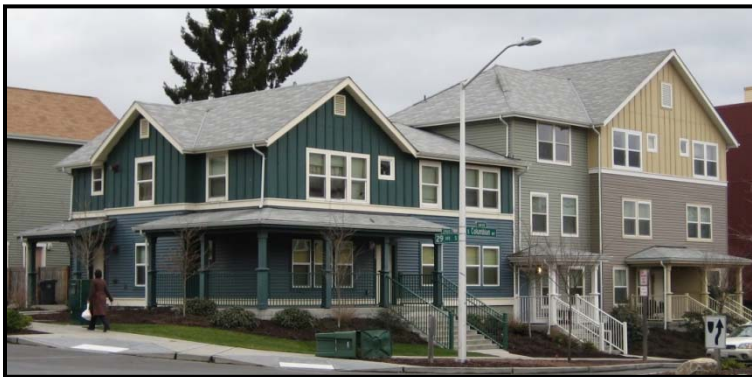
Figure 15.39.320F Example of vertical and horizontal changes in rooflines and variations in roof forms.
