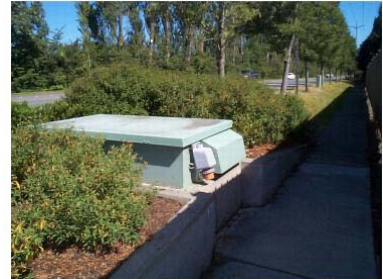
Access Concealed Through Grade
