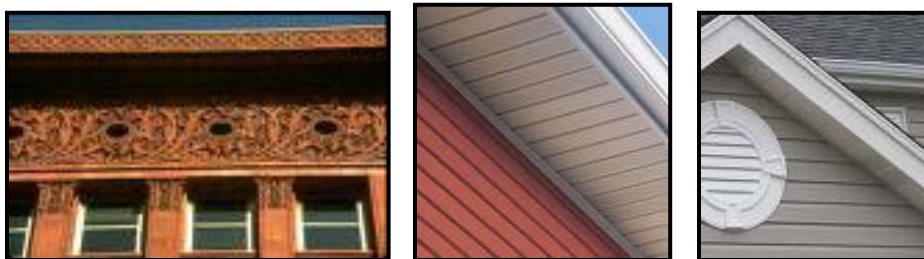
Figure 15.39.320K Examples of cornice, soffit and fascia details.
