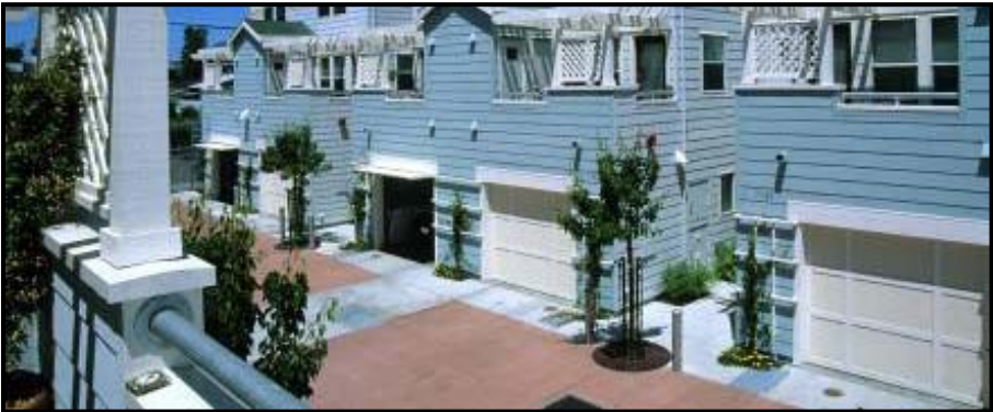
Figure 15.52539.240C Example of auto court constructed with scored and dyed concrete.
