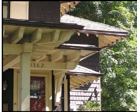
Figure 15.39.320I Example of rafter tails.
