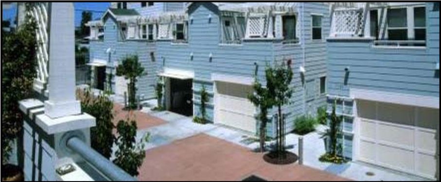
Figure 15.525.240C Example of auto court constructed with scored and dyed concrete.
