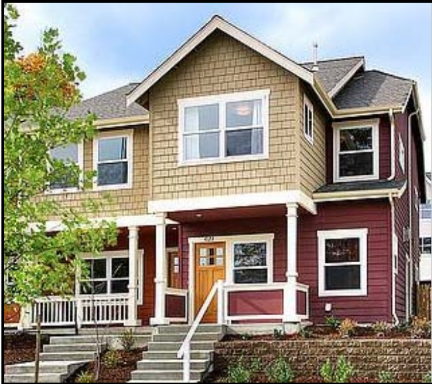
Figure 15.39.310A Clearly defined main entry with weather protection and various architectural design elements
