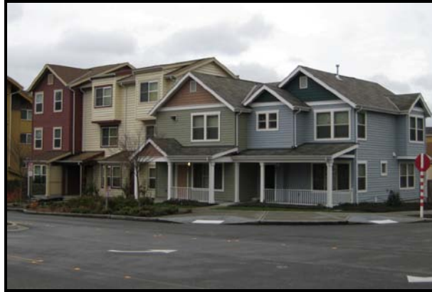
Figure 15.39.220A Example of units oriented to the street.
