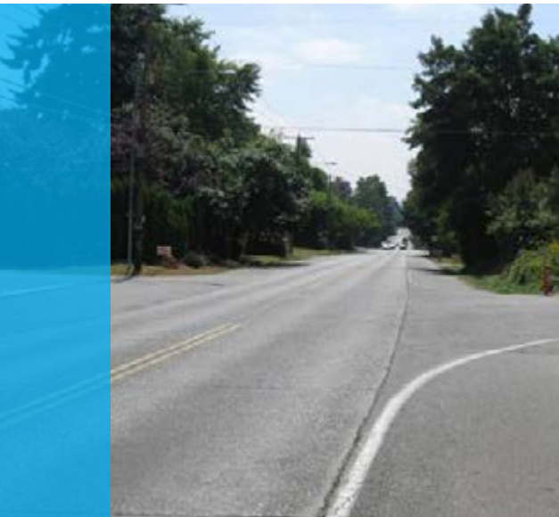
MILITARY ROAD S CONSTRUCTION - BEFORE
