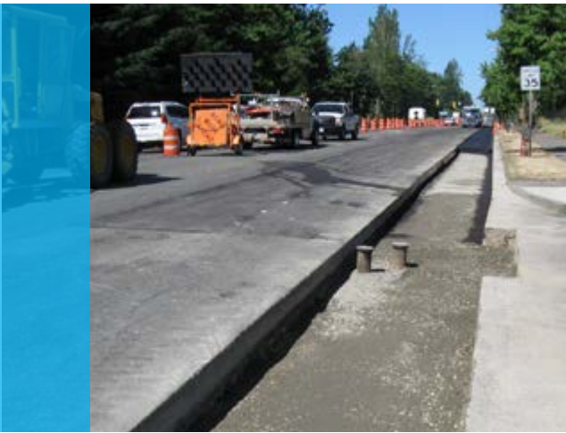
CONSTRUCTION ALONG S 168TH STREET
