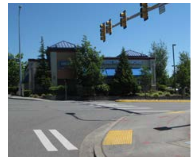
Existing curb ramps with truncated domes help direct pedestrians across the intersection.
