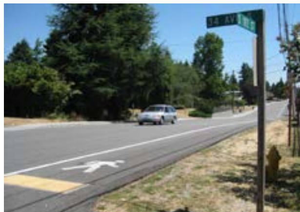
Existing paved shoulder walkway, a delineated pedestrian facility on a local street in SeaTac.
