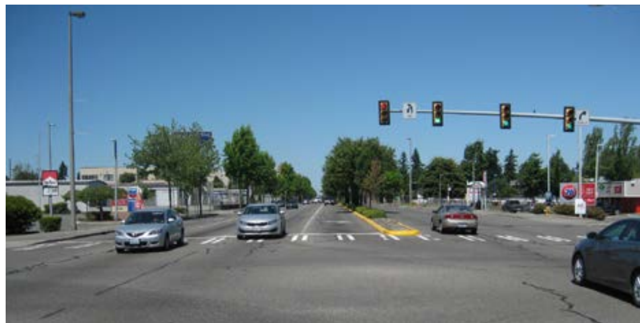
The intersection at International Boulevard and S 200th Street is seven lanes across. Signal timing should take pedestrian speeds into account.
