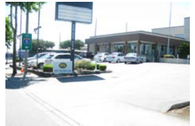
Parking lots separate the front doors of businesses from the street frontage.
