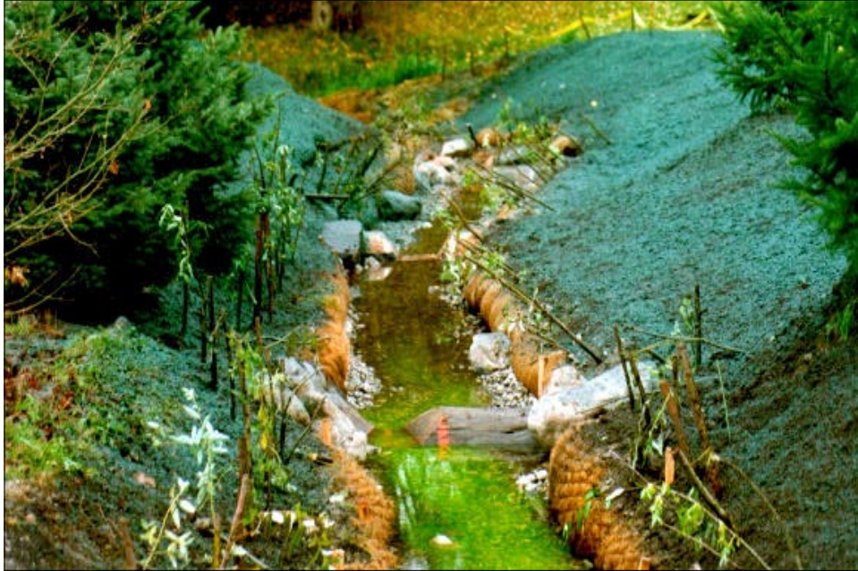
Coir logs used as habitat protection at the toe of a bank
