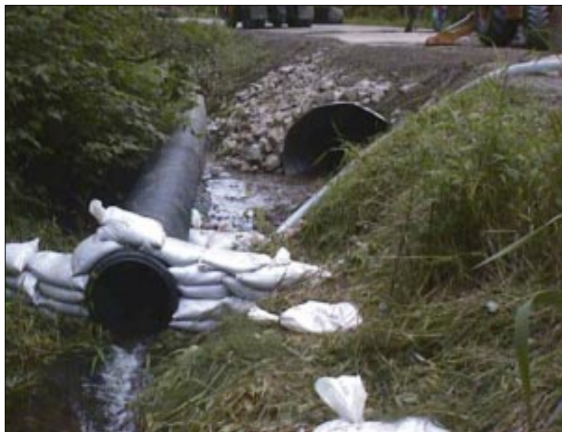
Sandbags holding bypass pipe in place and detaining sediment laden water on site
