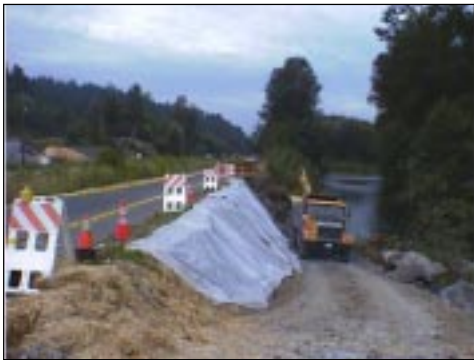
Plastic covering used as erosion protection on a slope at construction/repair area. Note additional use of mulch in area
