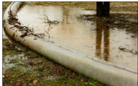
Continuous berm intercepting water from construction area
