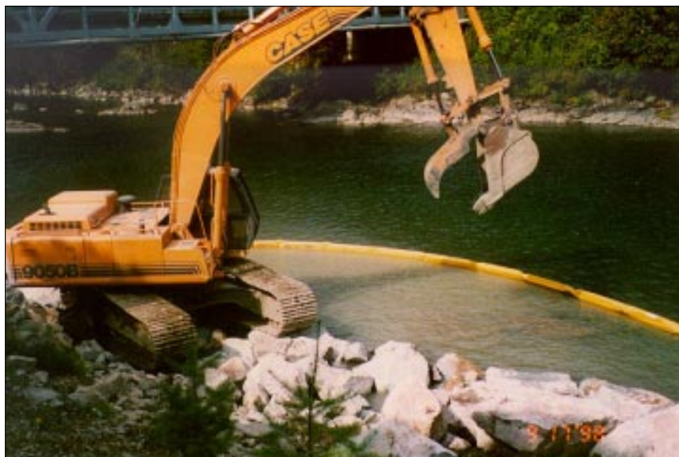
A river repair project in progress using a turbidity curtain to contain turbid water
