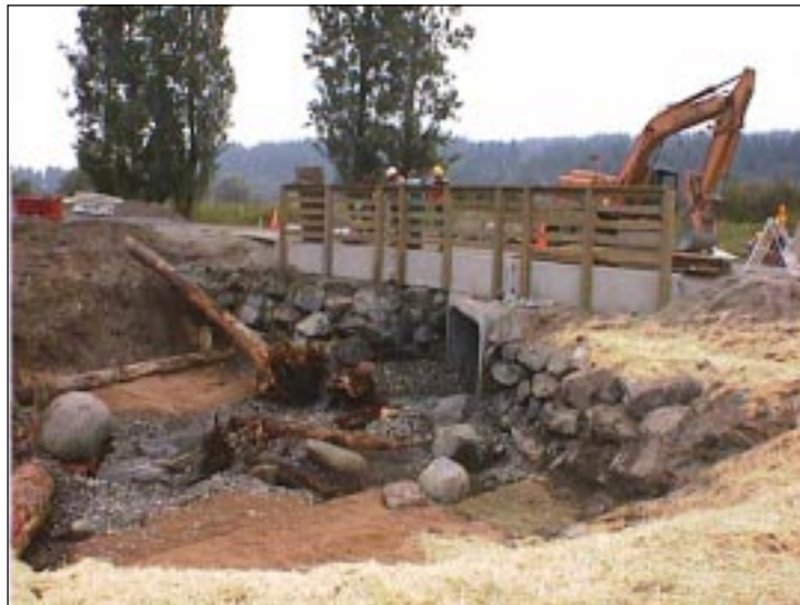
Large woody material placed in streambed to provide fish refuge. Note use of streambed gravel, mulch, and coir fabric
