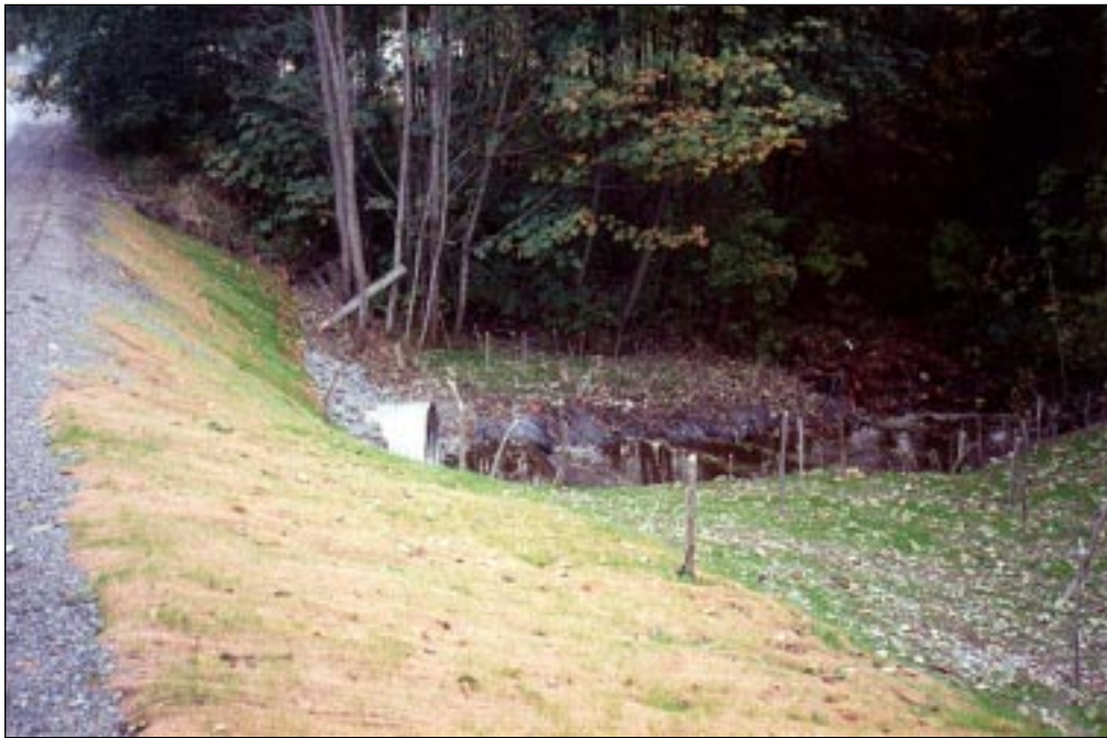
Using straw and live staking to reduce erosion and provide vegetative cover once vegetation has established
