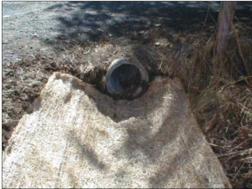
Silt mat installed in ditch to decrease erosion and allow settlement of suspended solids
