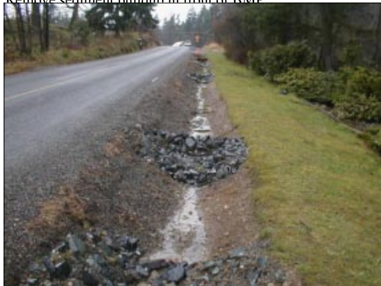
Rock check dam in ditch to provide reduction in water velocity
