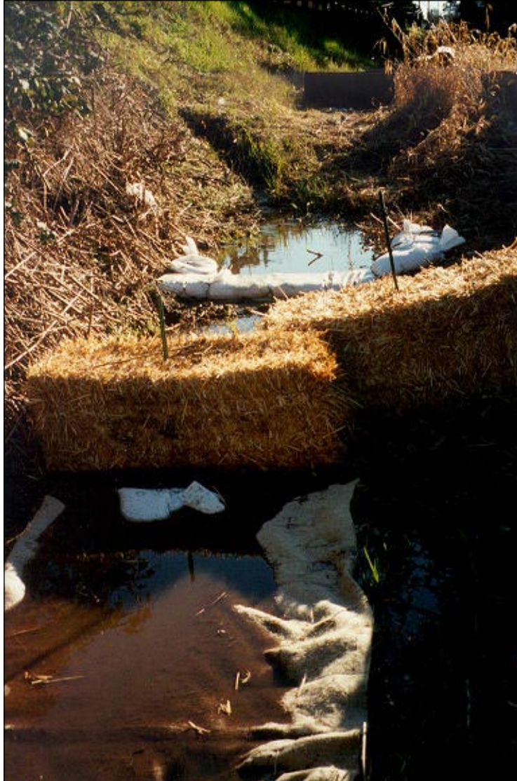
Straw Bale Barrier (2) reducing water velocity and erosive forces. Note other BMPs also being used
