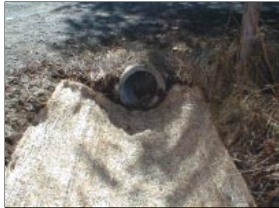
Lining a ditch with soil stabilization matting to reduce erosion
