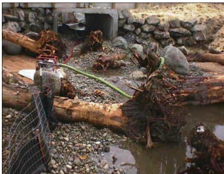
Large woody debris placed in streambed to provide salmonid refuge. Note use of streambed gravel, dewatering with pump, and mulching
