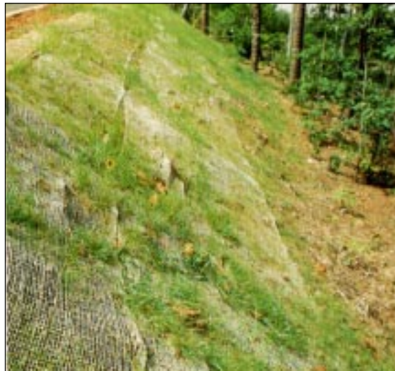
Stabilizing the soil using matting and hydroseeding
