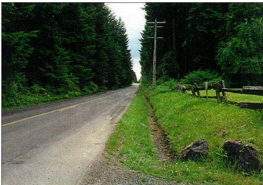
Roadside ditch with a vegetative buffer
