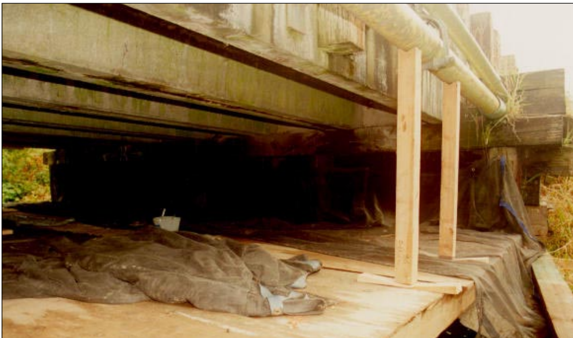
Plywood work platform providing a safe work environment and containing fallen debris from entering water during construction, maintenance, and repair activities
