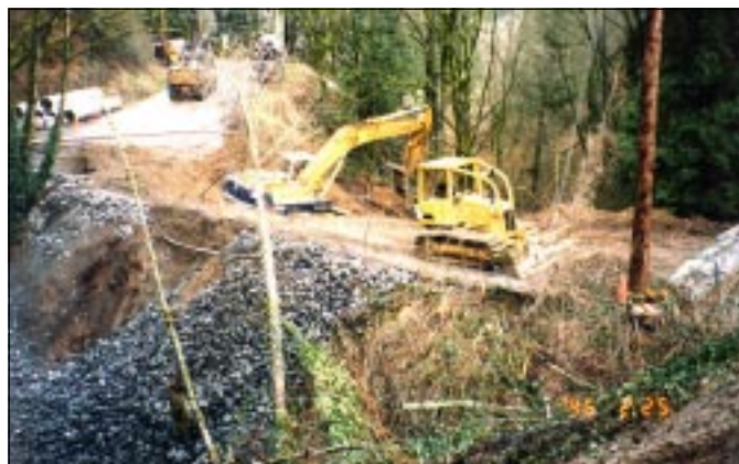
Rip rap used to provide bank stability
