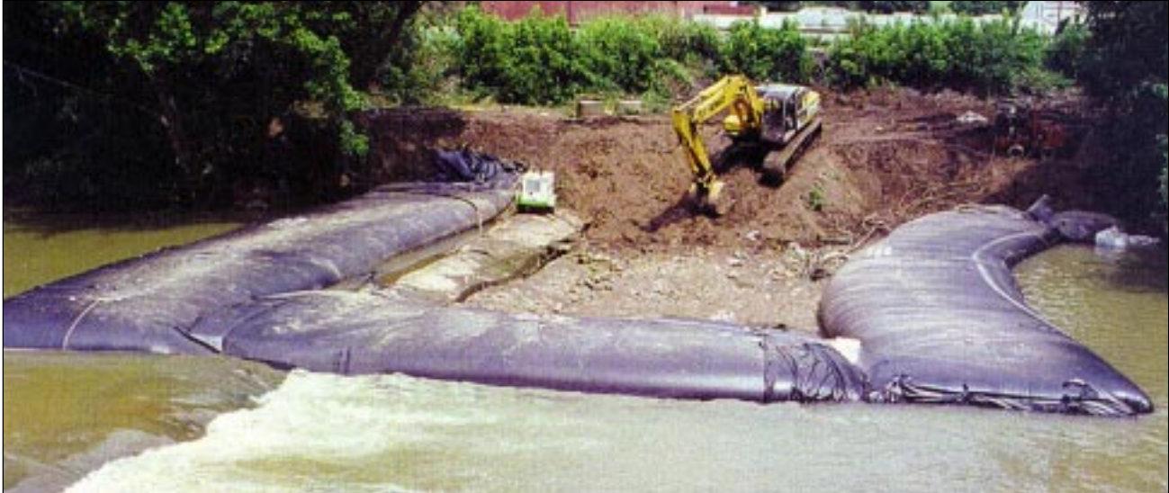
Aqua barrier used as coffer dam
