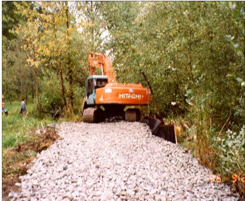
Access road installation
