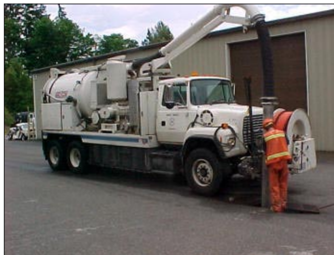
Vactor truck removing sediment from catch basin
