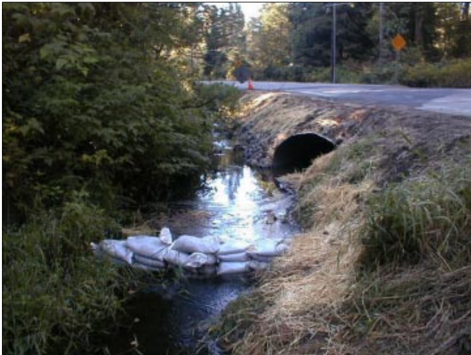
Sandbags used as a cofferdam
