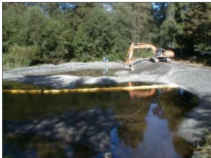
Large silt pond with turbidity curtain in place
