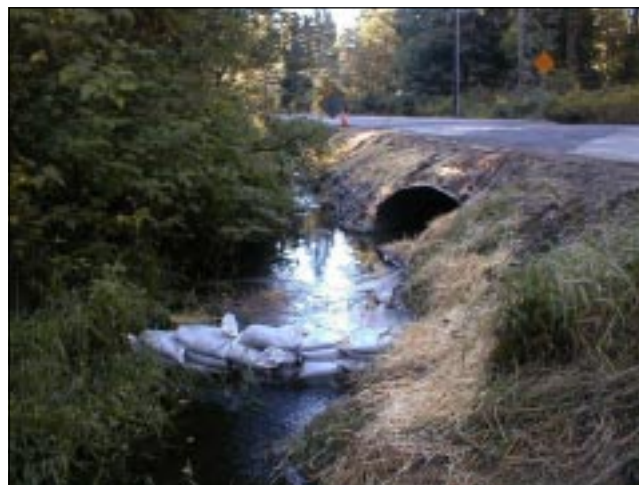
Sandbags acting as a barrier
