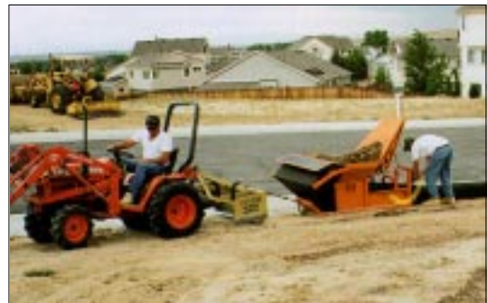
Continuous berm retaining soil particles and debris
